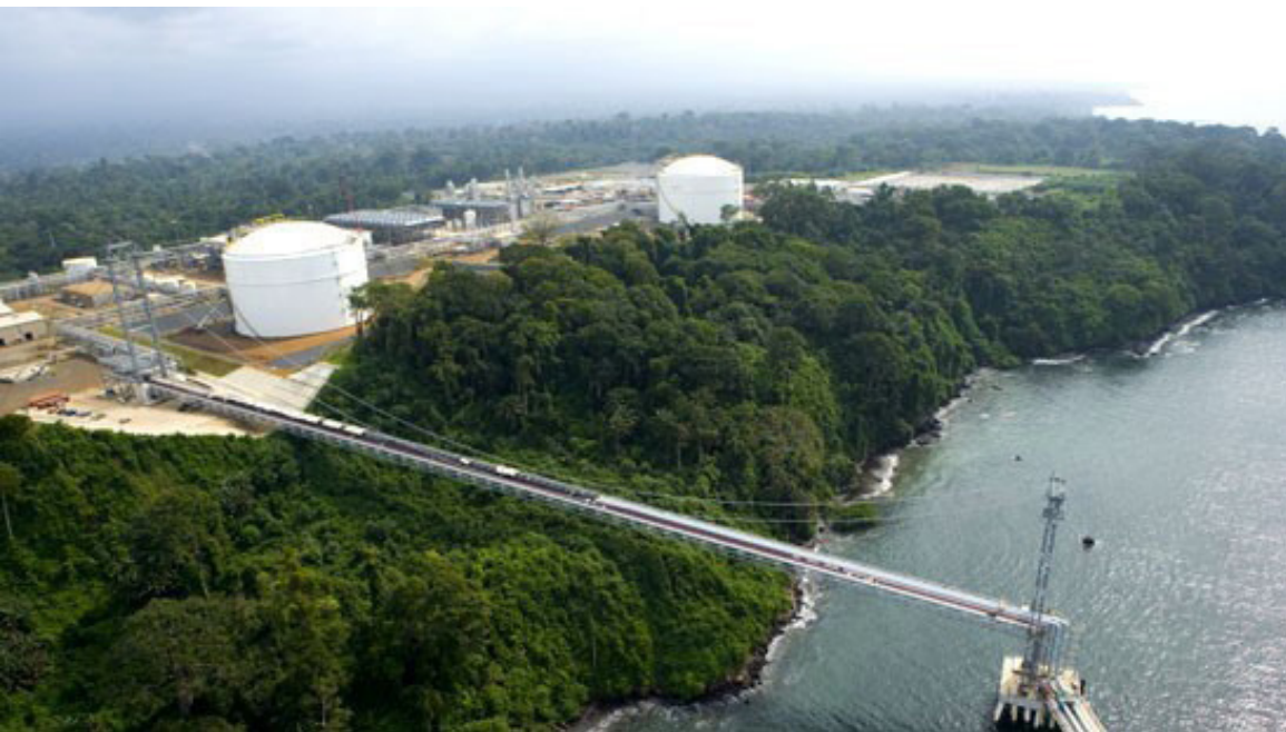
Figure 13: Offloading Jetty for Equatorial Guinea
